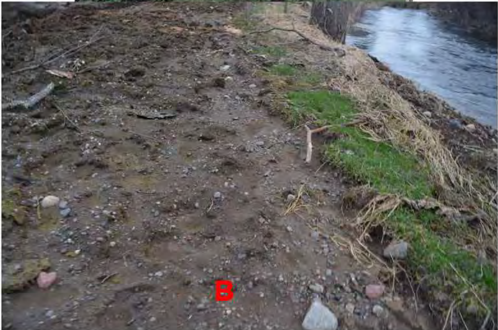
Foytik FP-10 Runway: Eroded, washed gravel direct conduit
