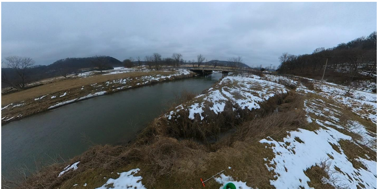
Image 8.2 – Chute 8: Severe undercut with slump and vegetative overhang
