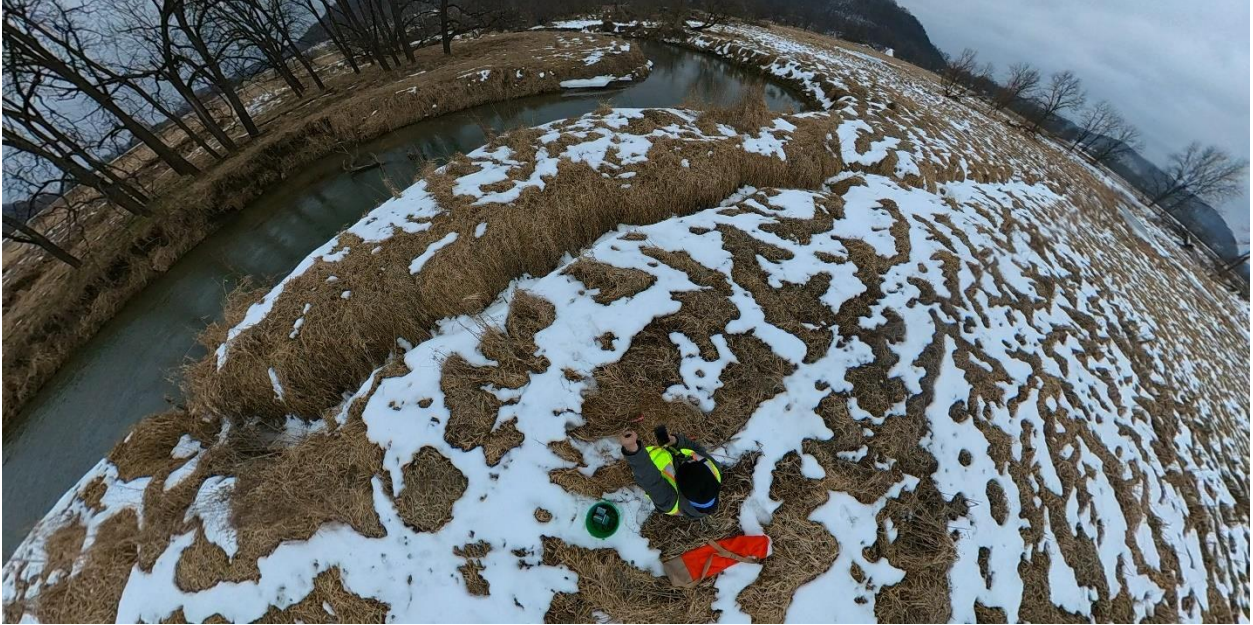
Image 3.0 – Chute 3: Moderate undercut with vegetative overhang
