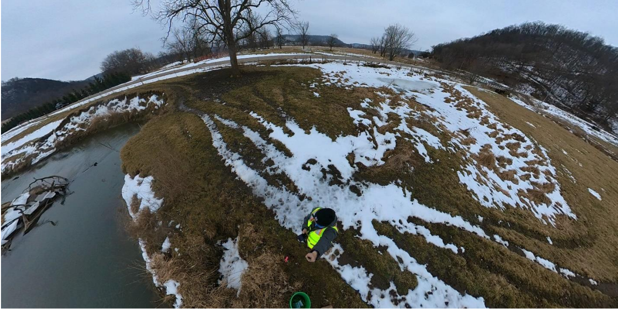
Image 7.1 – Chute 7: Moderate undercut with slump and vegetative overhang
