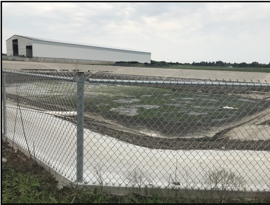
Photo 14 (left): Looking south east from the north west corner of the process wastewater storage that is used for leachate and feed storage runoff. A white post (pictured left) can be seen along the north wall of the storage near the outlet pipe which contains permanent markers. A safety fence was also observed around the entire perimeter of the storage.
