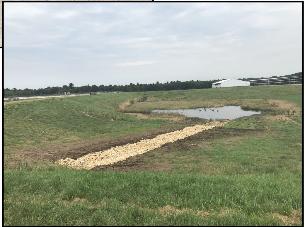
Photo 6 (right): Looking north across the storm water basin that can be used as secondary containment in the event of an emergency with WSF 1 or WSF 2.
