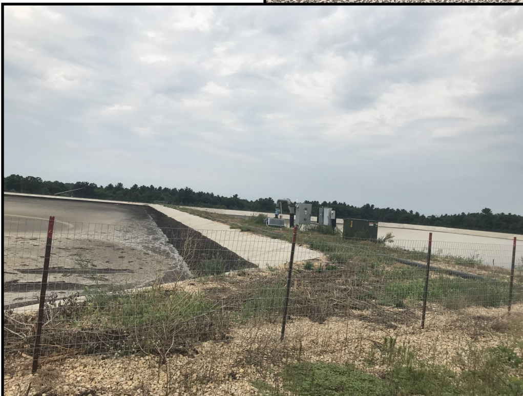
Photo 4 (bottom left): Looking west at the pump out tank between WSF 1 and WSF 2. The pump tank transfers the contents of each storage to the load station located at the south east corner of WSF 1 (pictured in photo 2) to be land applied.
