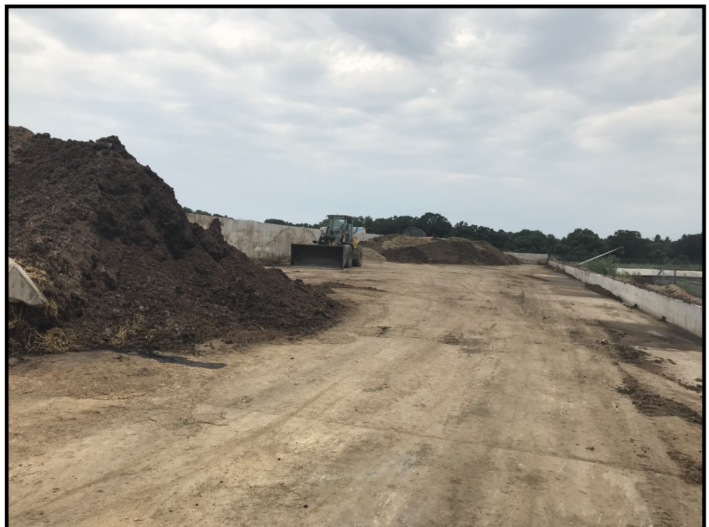
Photo 22 (right): Looking west across the concrete solid stacking pad where animal mortalities are composted. Mortality compost material can be seen pictured left.
