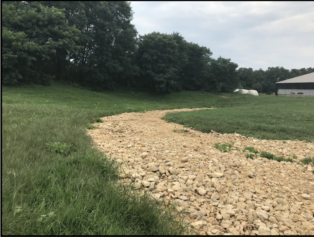
Photo 23 (left): Looking at the storm water conveyance at the west end of the site just south of the abandoned calf hutch area and former calf barn. The operation has addressed past erosion issues in this area and have placed rock within the flow path to prevent future erosion.
