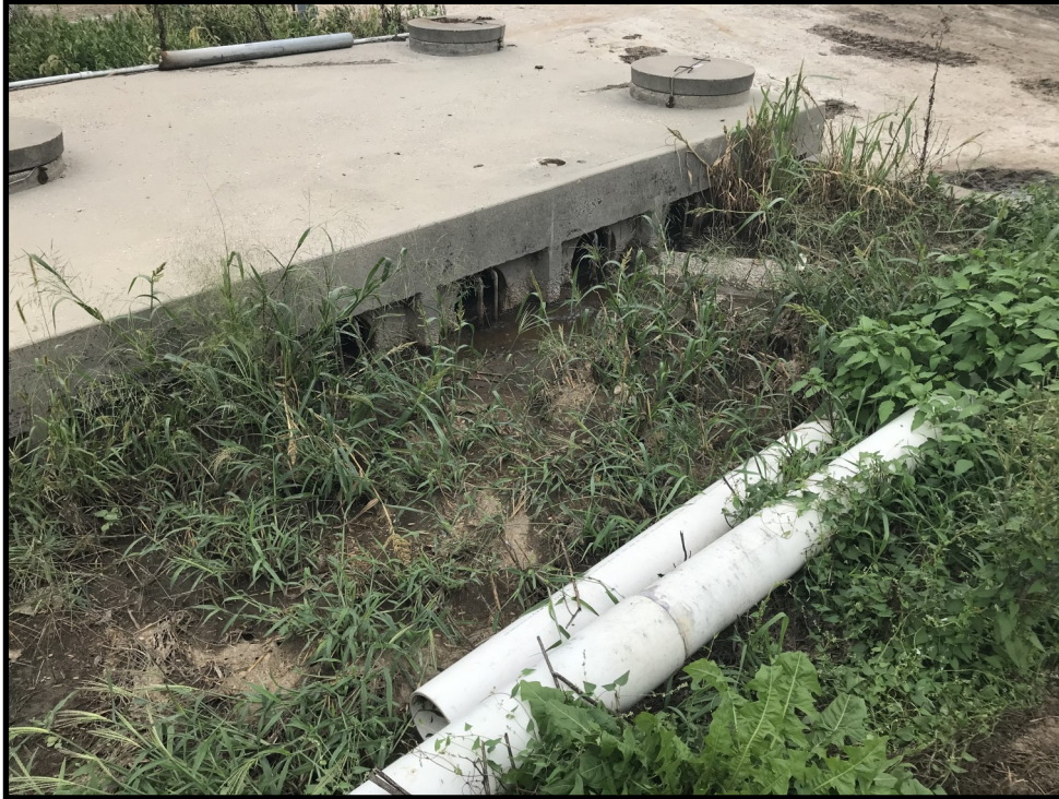
Photo 16 (left): Looking at the first flush collection tank that was installed as part of the runoff control system when the feed storage area was first constructed. The contents of the tank are now pumped to WSF 1 as needed. A considerable amount of vegetation and debris was observed around the tank inlets.
