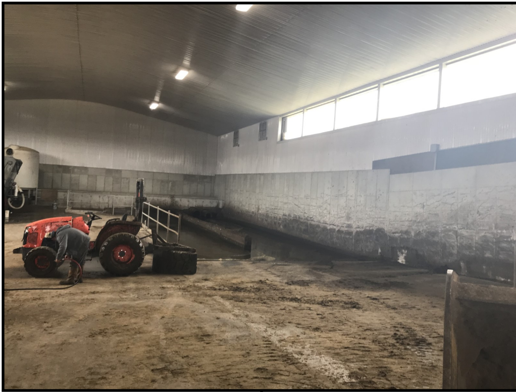
Photo 10 (left): Looking at the manure transfer lanes within the solids separation building. All liquid manure generated by the operation is transferred to the solids separation building. After manure solids are separated out, remaining liquids are transferred to WSF 1 or WSF 2.
