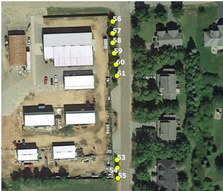
Figure 10. Ash street trees on Swan Ave.
