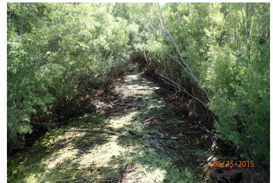
Debris on Dutchman Creek downstream Overland Road.
