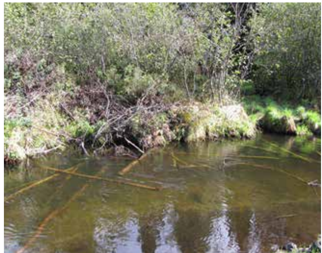
Evergreen River 2012 Project Area – channel shaping and tree/rootwads installed.
