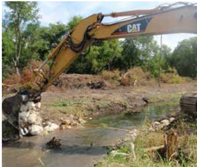
Bank stabilization and addition of woody habitat.
