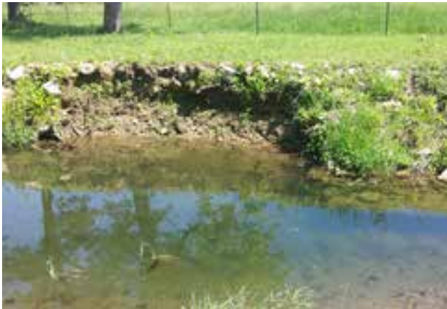
Creek 8-8 (Rundahl Creek) -Stream bank damaged by flood
