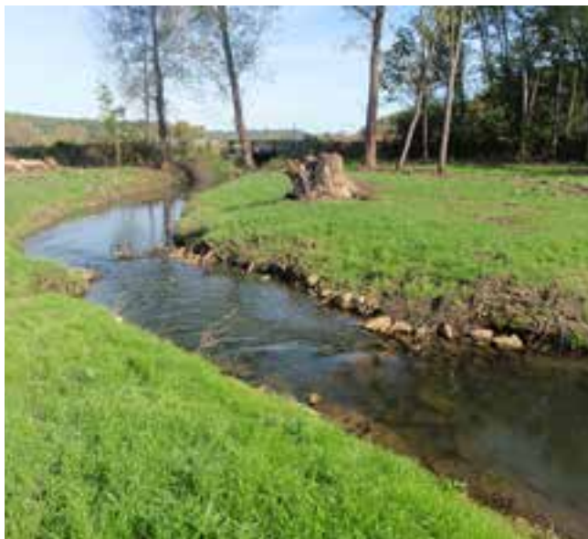
Finished bank with new seeding
