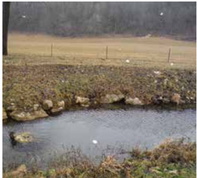
Creek 8-8 (Rundahl Creek) –Repaired stream bank damaged by flood
