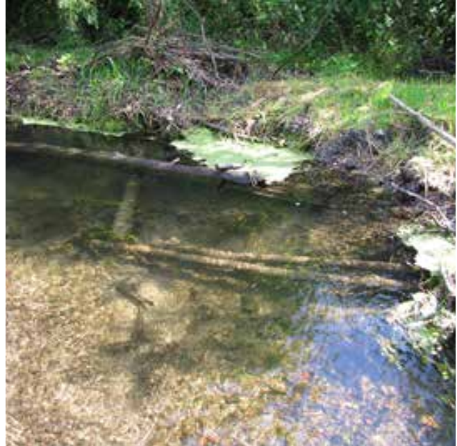
Spring Creek (Lincoln County) – channel shaping and log jam installation.
