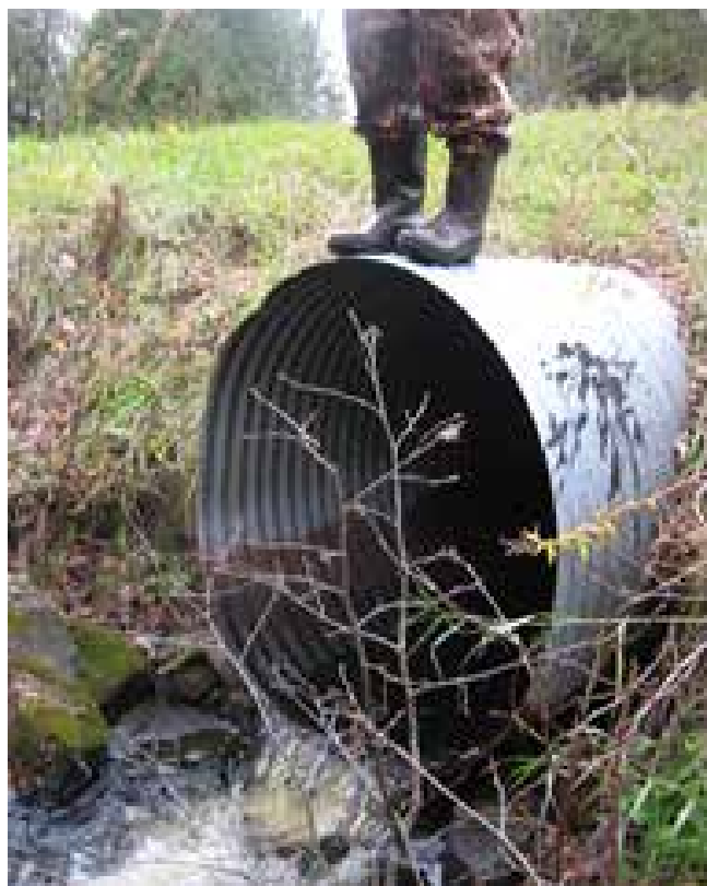
Perched outlet on McDonald Creek, a Class I trout stream.
