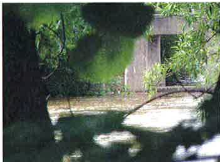
June 2008 storm event: water level is almost above top of gate and the same level upstream and downstream of the dam structure.
