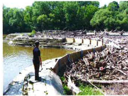
A picture of the serpentine spillway from 2010, undergoing some emergency repairs.
