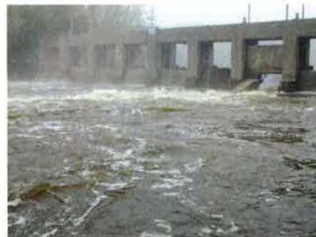
Estabrook Dam on May 11, 2004. Note only two gates were opened.
