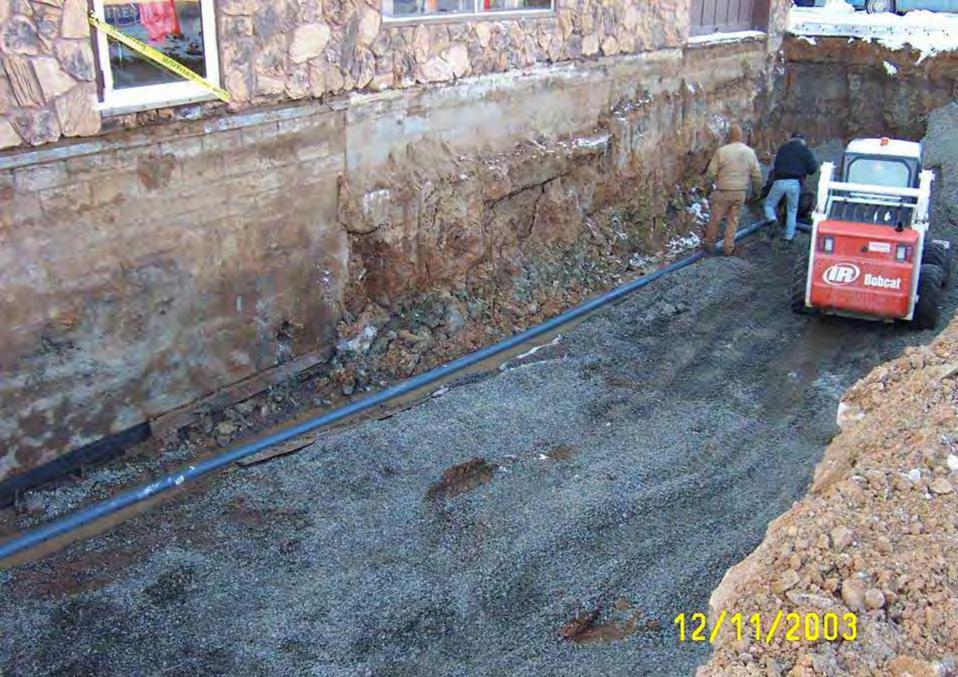
Installation of the depressurization system. Bottom tier.
