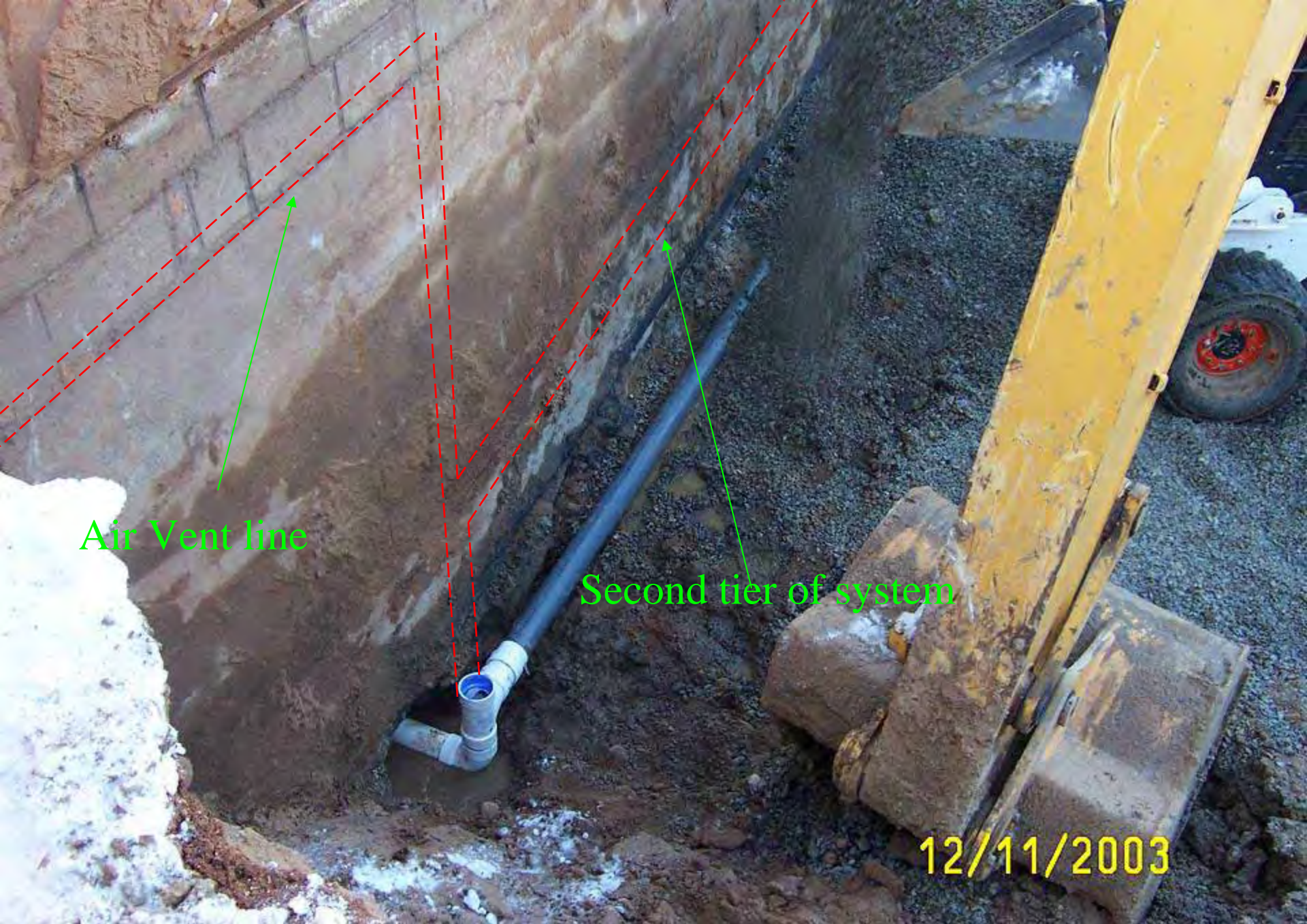
Depressurization system being tied into sump inside basement.
